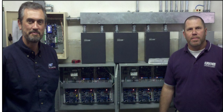
Francis Chapman of ASI Controls (left) and Ken Cooksey of PC Automation (right), with ASIC/1 VAV and Heat Pump controllers behind
